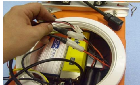
(Fig. 4.27) Connect instrument power leads to the batteries
